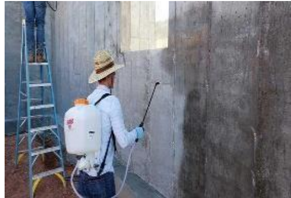
fig 5.3 water proofing spray
